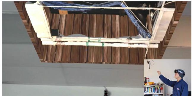
Displaying virtual excavations to facilitate building maintenance.
